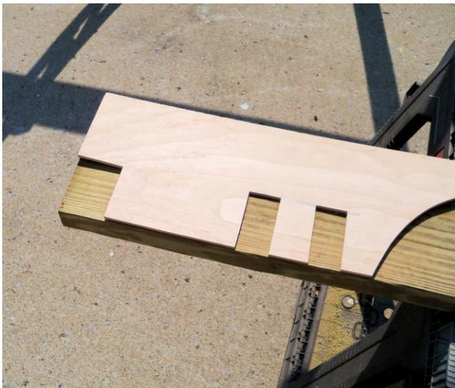
The 'arches' are connected by the 8 foot long upper beams. Four of these needed to be prepared before setting the uprights. The template was again used. Each upper beam got one end with the decorative cut and two notches to fit over the cross beams. The other end got a simple notch to overlap the center cross beams.
