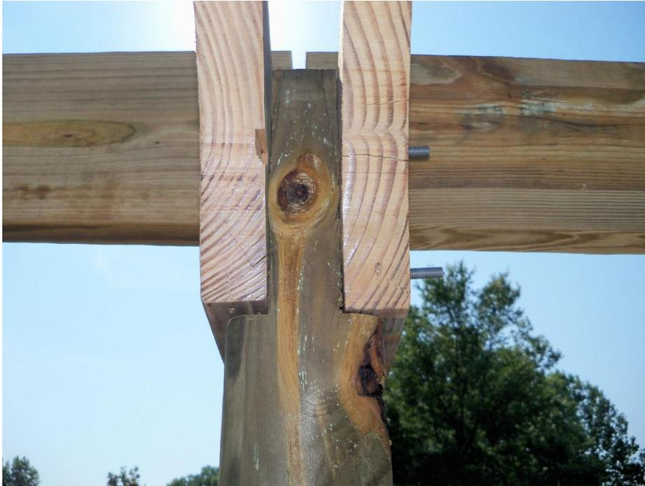
Step one was preparing the posts. I notched two faces of the 4x4's to provide a shoulder for the cross beams to sit on.
